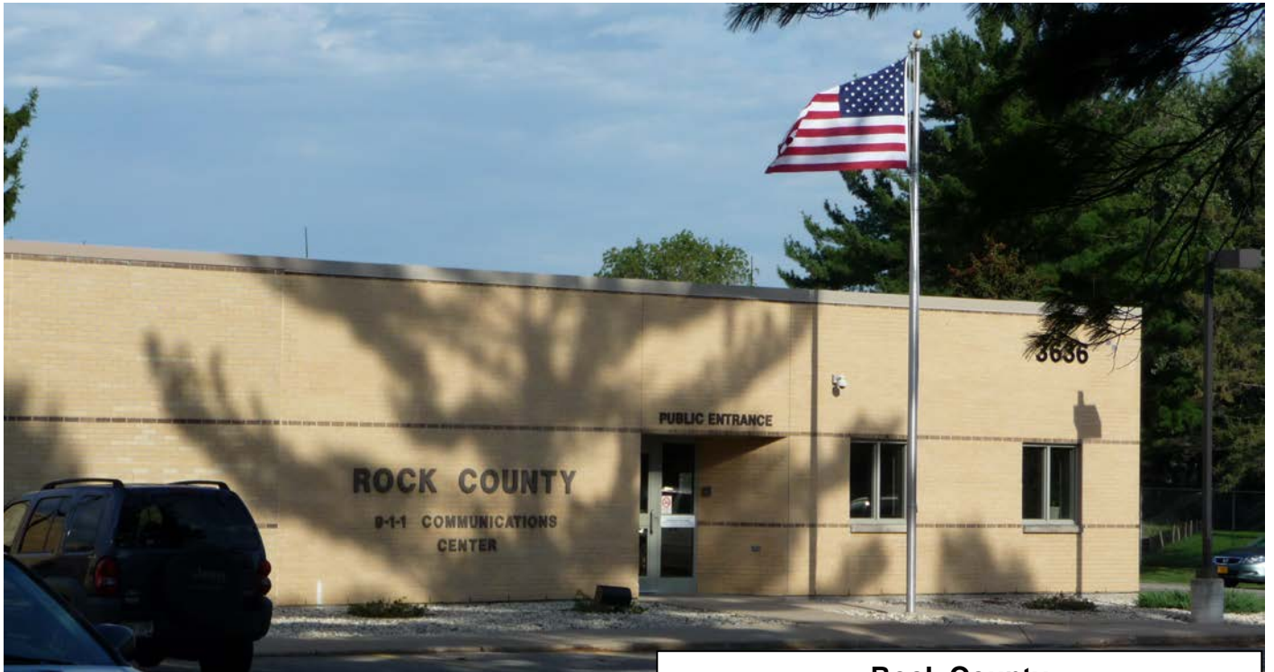
Rock County 911 Communications Center Expansion Janesville, Wisconsin Potter Lawson, Inc., Architects
